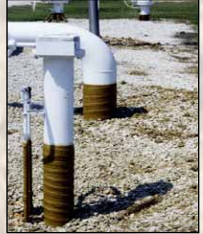
Transition zone of large pipeline
