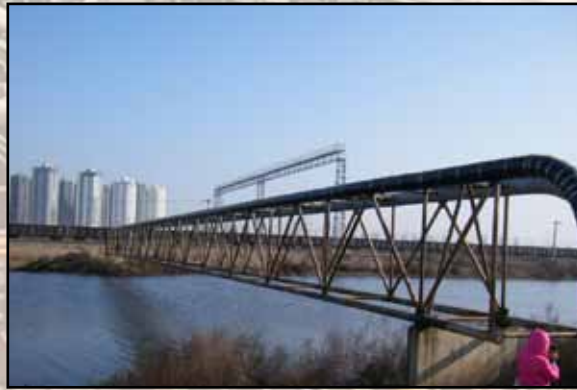
Insulated pipeline across bridge
