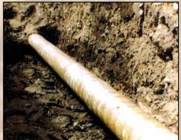
Below ground pipeline can be backfilled immediately
