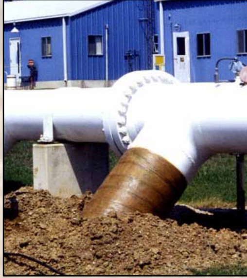
Transition zone of large pipeline
