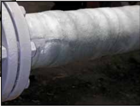
Tape cut for section and repair
