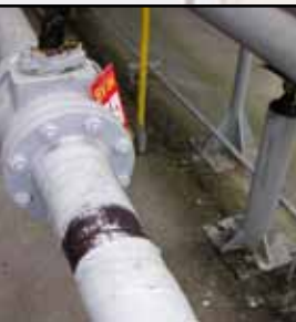
Tape cut for section and repair
