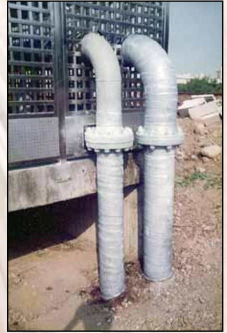
Pipeline soil transitions
