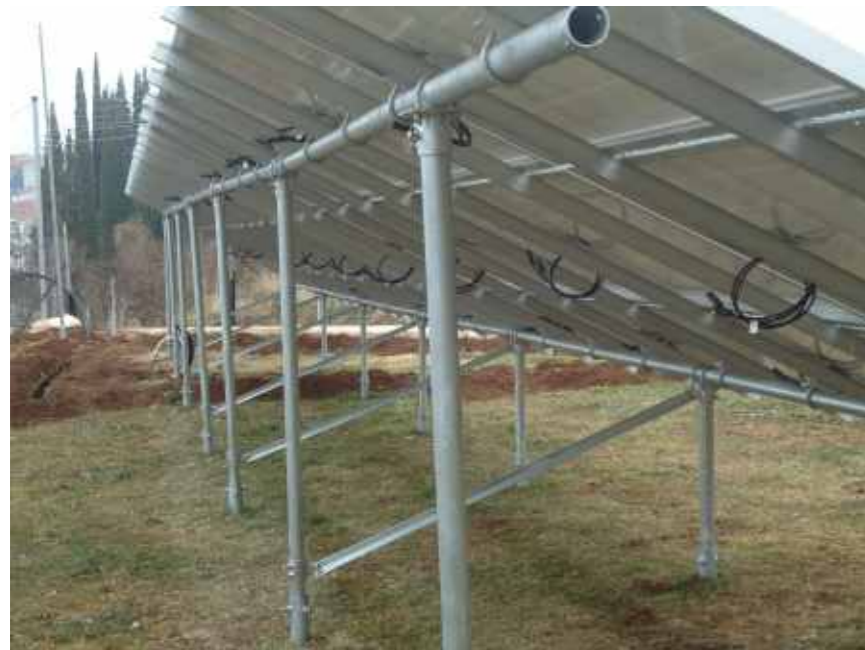
UB Ground Mounting installed on Ground Screw 68x1000
